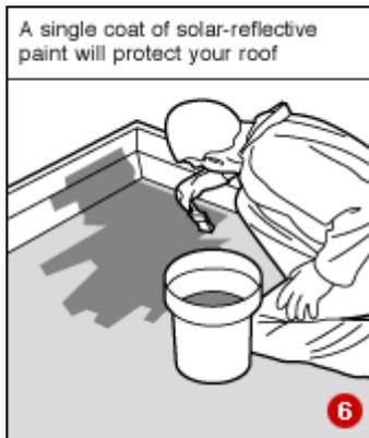
Dark-coloured felt will attract a great deal of heat in the summer and if the flat roof has insulation underneath, the temperature can only escape upwards. To counteract this white stone chippings are often used to reflect the sun. The problem with chippings however, is that if anyone walks on the roof, the chippings can get pressed through the felt and
